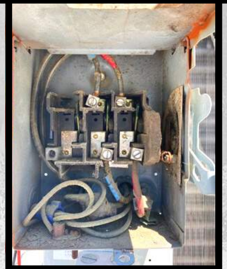
UNSAFE DISCONNECT THAT HAS BEEN BYPASSED
